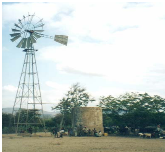
Figure 14: Wind Pump Supplying Water to Kisigisa Village in Kongwa District, Tanzania
