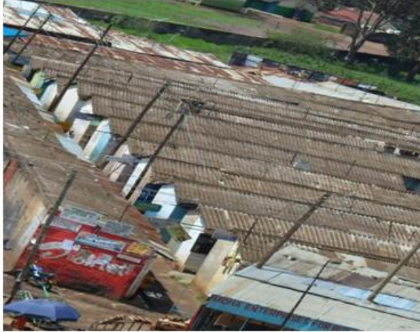
Some of the legal electricity connections in Kibera slum
