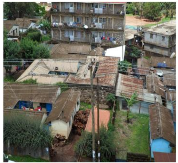
Overhead power by Kenya Power
