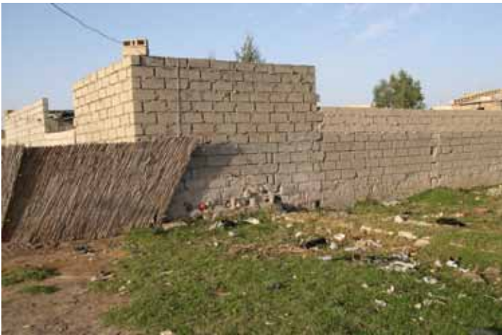
Figure 7. Example of suspended illegal connections in Ben-barack
