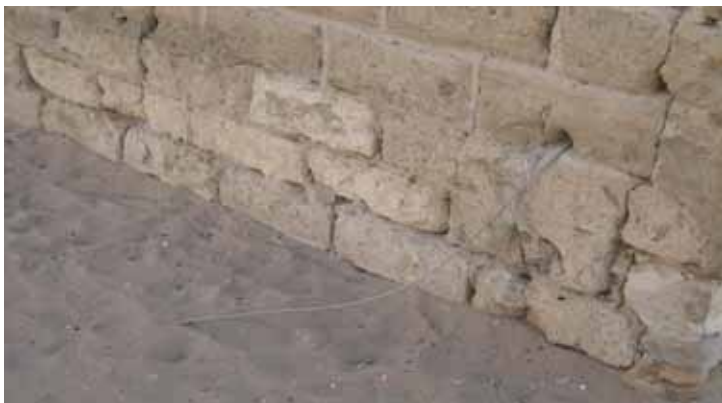
Figure 5. Example of underground illegal connections in Ben-barack
